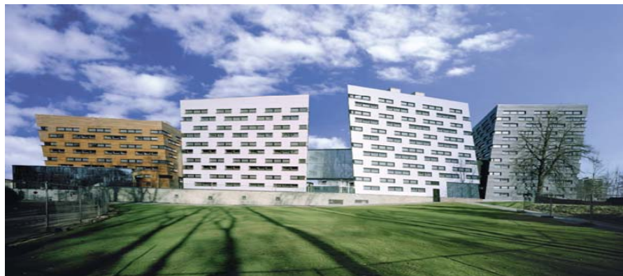
Business Center on Passive House Standard
